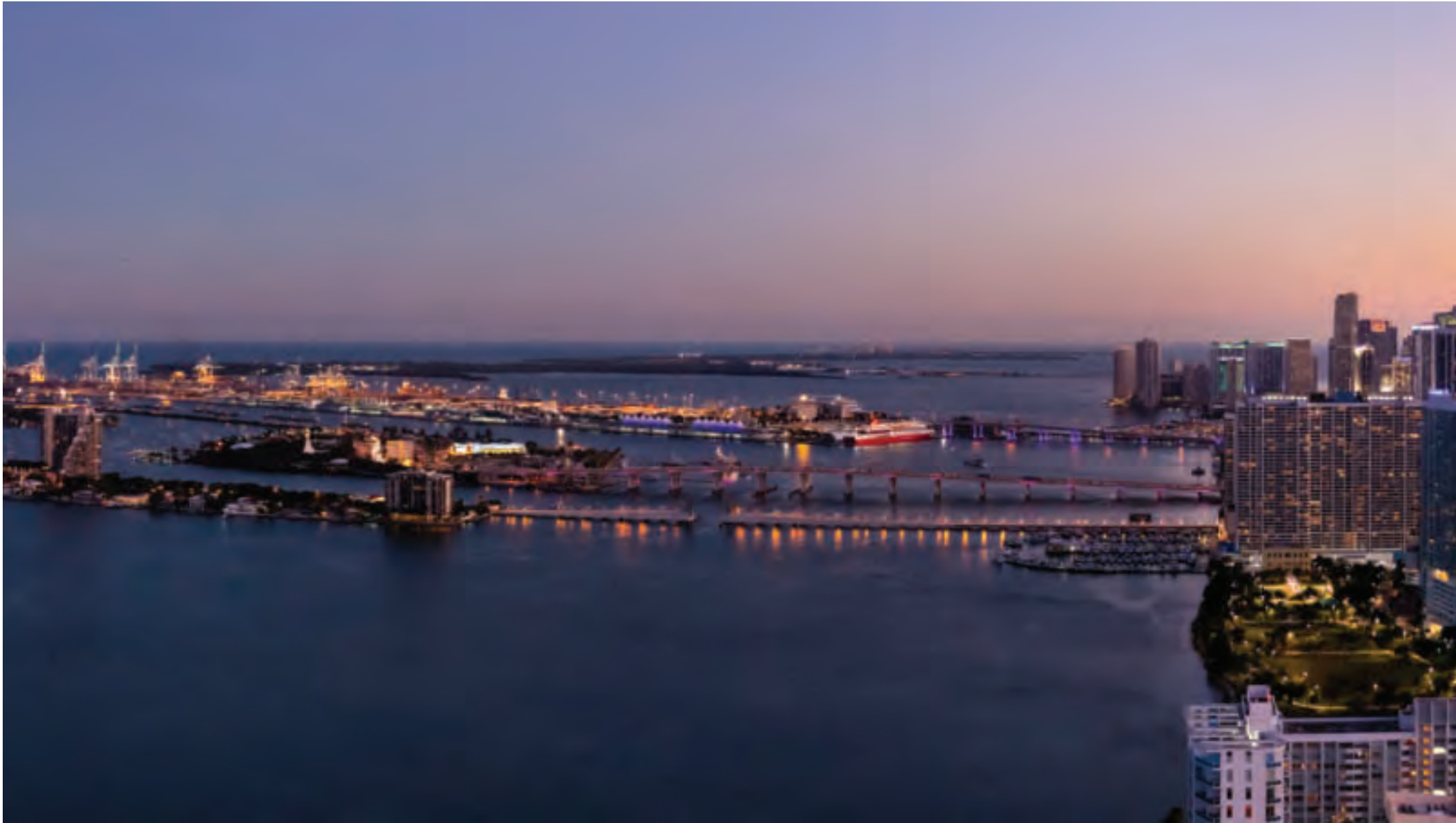
VIEWS EAST AND SOUTH OVERLOOKING THE VENETIAN CAUSEWAY, DOWNTOWN MIAMI, AND THE ATLANTIC OCEAN
